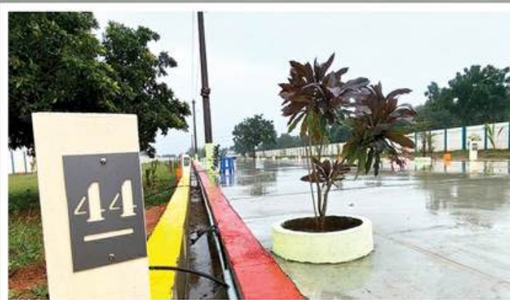
Well-Planned Storm Water Drainage & Street Lighting Facilities
